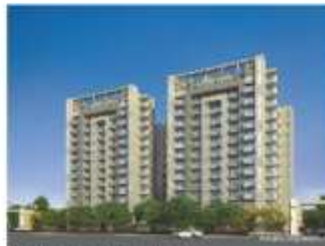
PLATINA, GURGAON Luxury Group Housing Project
